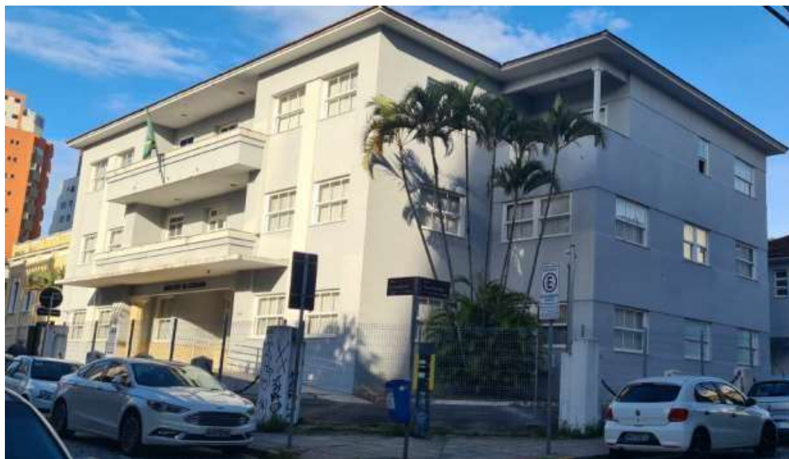
Figura 2: SRA/SC – Bloco A – fachada principal
