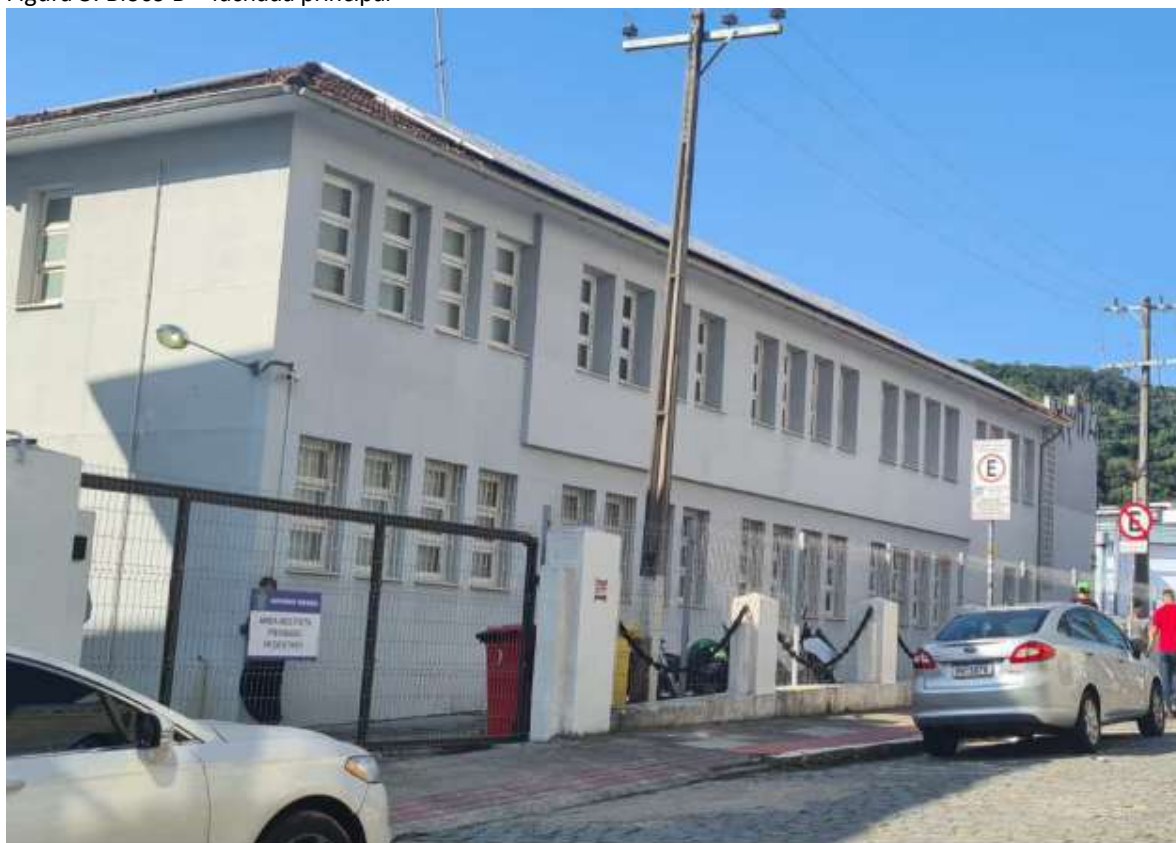
Figura 3: Bloco B – fachada principal
